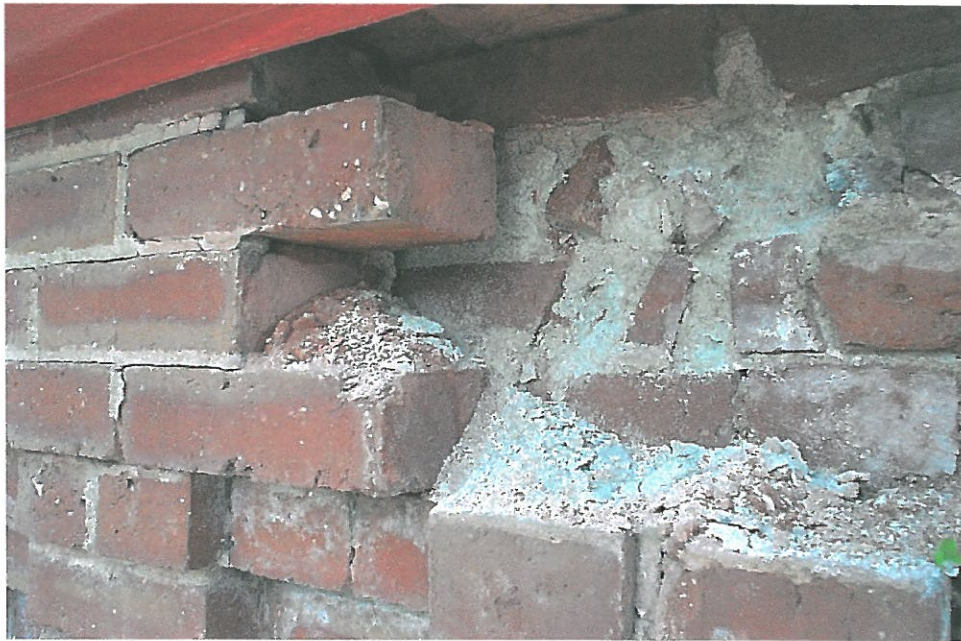
Mortar disintegration.
