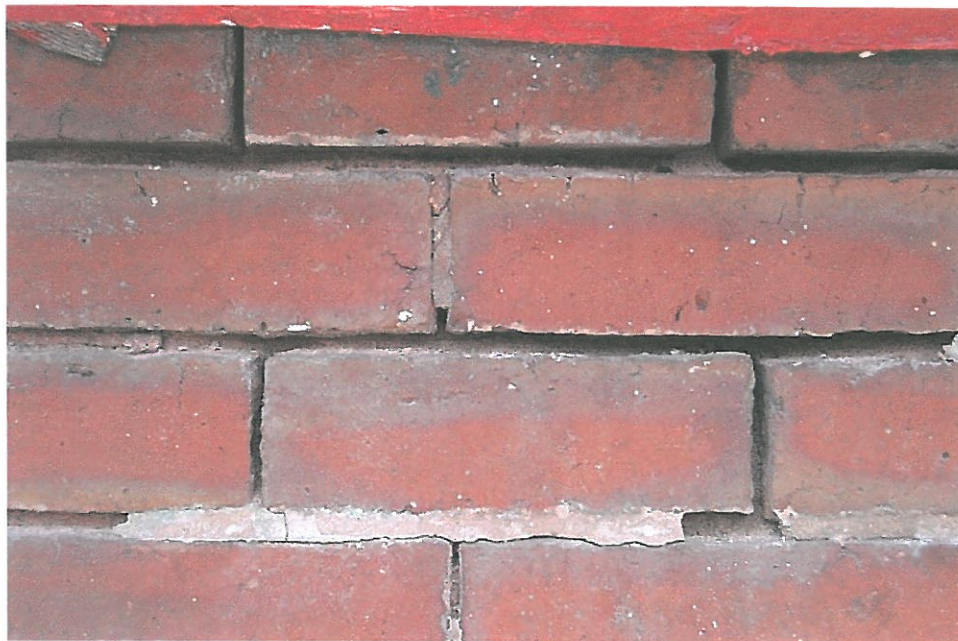
Missing mortar typical of original walls.
