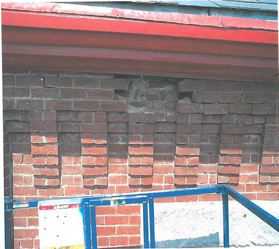
Wall deterioration at east wall
