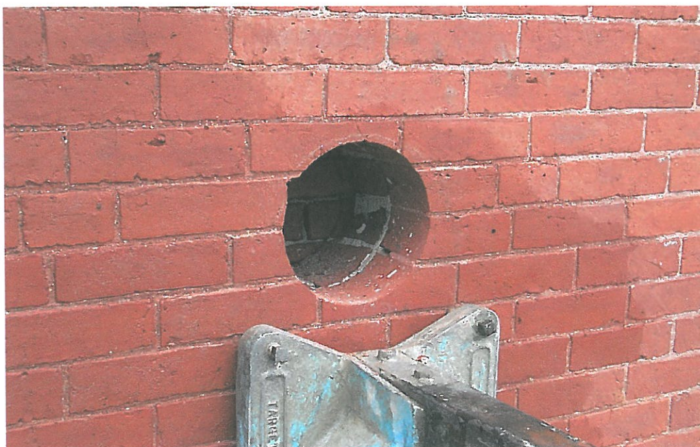
Brick core at wall base. Note good mortar condition.
