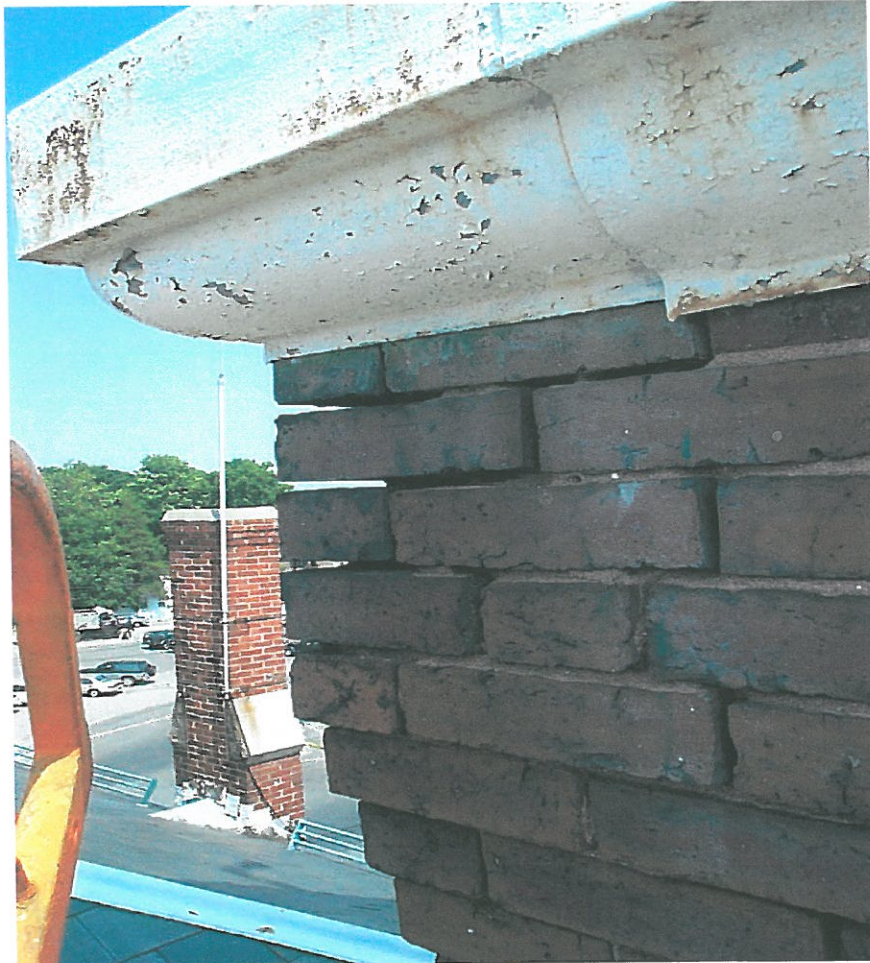
Wall deterioration at hose tower
