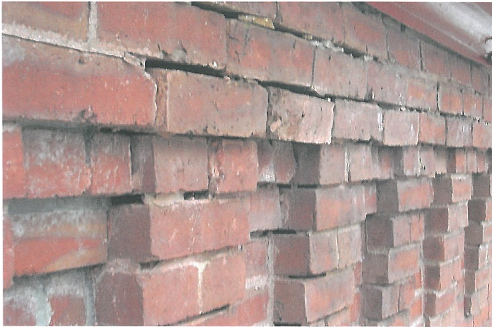
Dentil corbelling deterioration.
